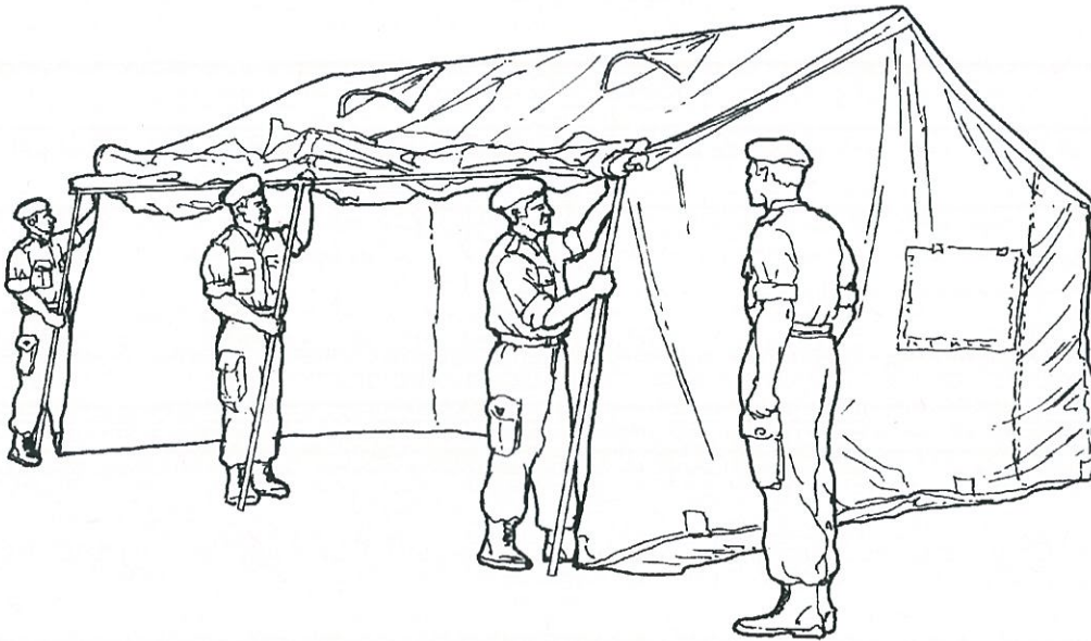
Fig 5-15 — Fitting Wall Supports To Eave Line
